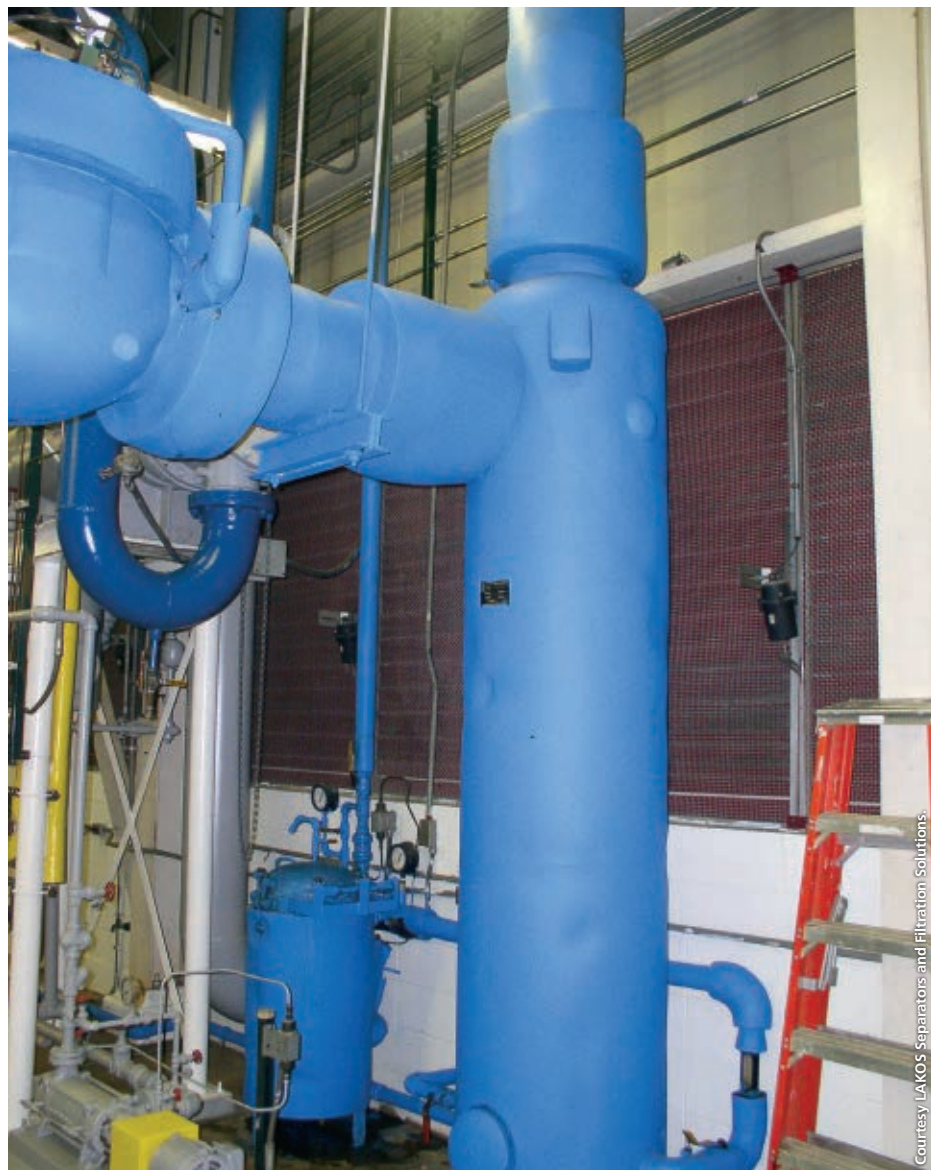
At Citizens Thermal's West Street Plant, the LAKOS RTS-1209B separator and CRS-836 closed recovery vessel have been providing filtration since 1992.
