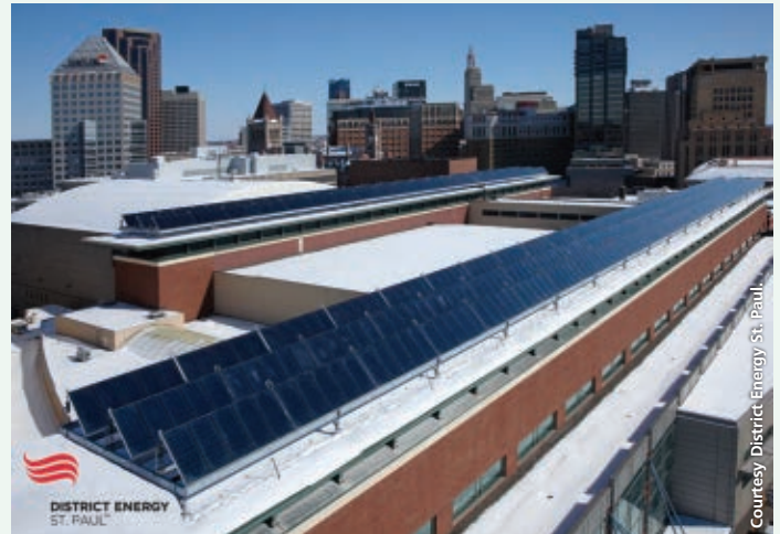
An installation of 144 solar panels atop Saint Paul RiverCentre generates 4.09 MMBtu/hr of thermal energy annually that is used at the convention center and by District Energy St. Paul.
