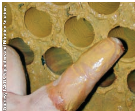
Filtration of a district energy system's water supply can prevent the buildup of unwanted contaminants, such as in these dirty chiller tubes.
