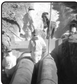
NATIONAL CENTER THERAPEUTICS MANUFACTURING - TEXAS A&M 24" HDPE CWSR INSULATED WITH GILSULATE®500XR. A&M'S CAMPUS DISTRIBUTION MASTER PLAN FOR CWSR/HWSR RECENTLY CHANGED FROM PIP TO GILSULATE®500XR.
