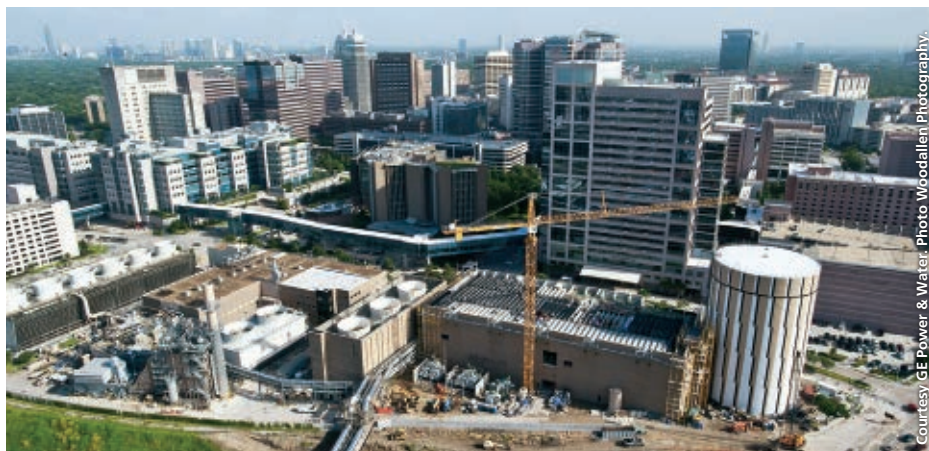
TECO's Central Plant site was under construction from 2008 until early May 2011. Nine months of construction remained when this aerial image with the Texas Medical Center campus in the background was captured. The expanded district energy facility's design allows TECO's capacity to reach 100 MW of on-site power generation, 168,000 tons of chilled water, 152,000 ton-hr of chilled-water storage and 940,000 lb/hr of steam.
