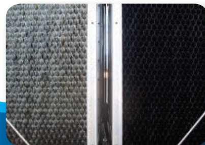
Cooling Tower Fill Before/After Cleaning
