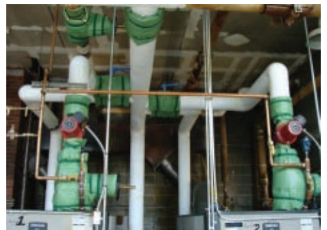
Pipe Fitting Components Insulated with Cut 'n Wrap
