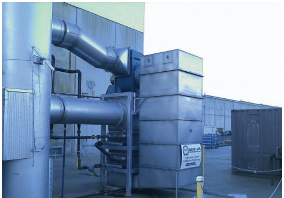
Del Monte Foods' Super Boiler flue gas condensing heat exchanger has a boiler fuel-to-steam efficiency exceeding 93 percent.
