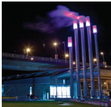
The Neighbourhood Energy Utility plant's flue stacks have been sculptured in the shape of a stainless steel hand. The fingernails, made from LED panels, change color depending on the amount of green energy being used.
