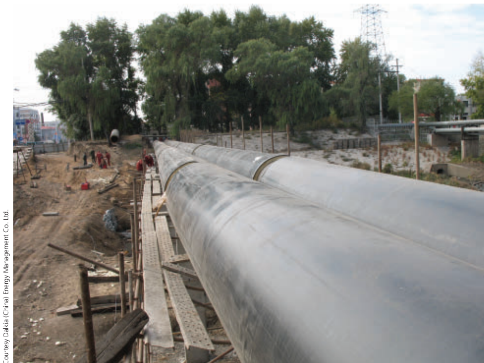
Pipeline for the north feeder was laid in 2009, crossing over a small river.
