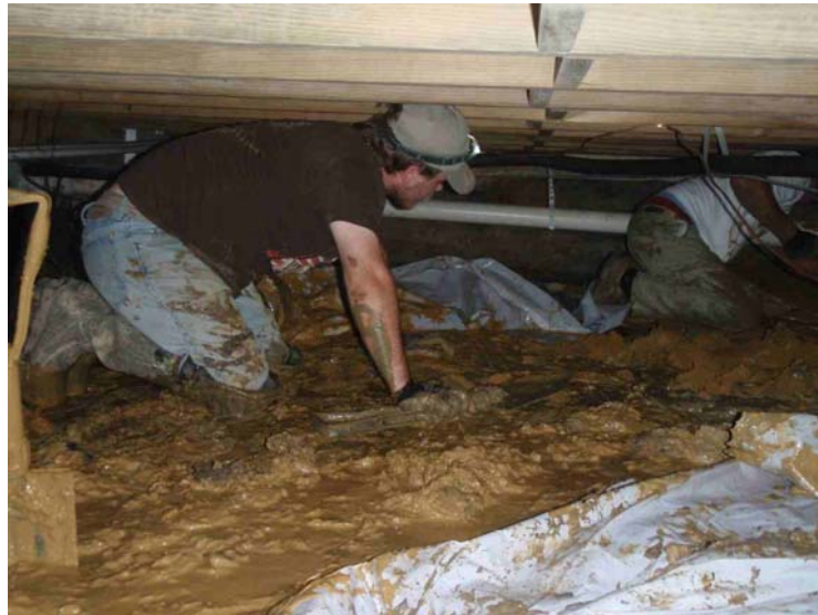
Home Crawl Space Insulation Davis' Home
