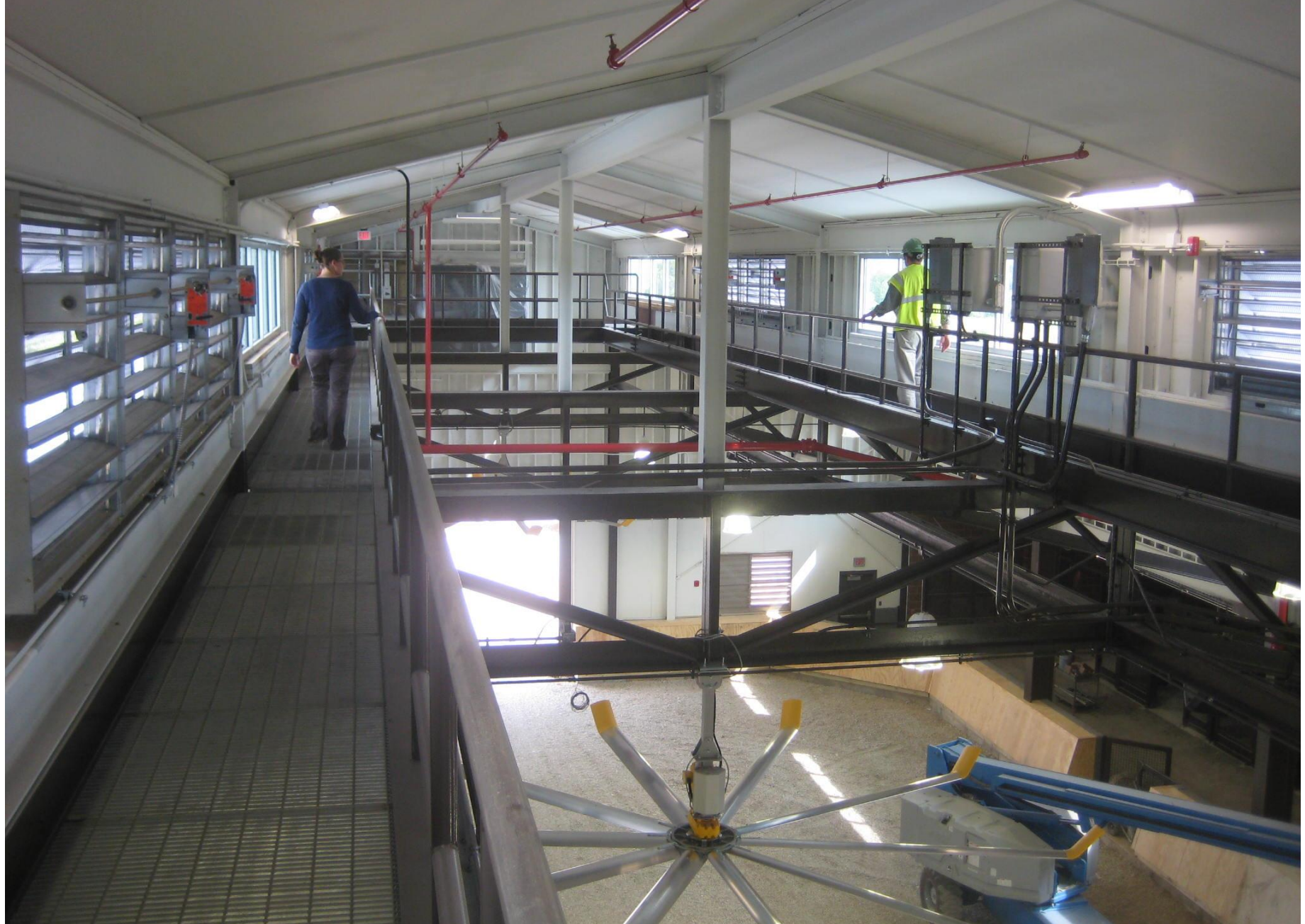
Arena - Ventilation & Daylighting
