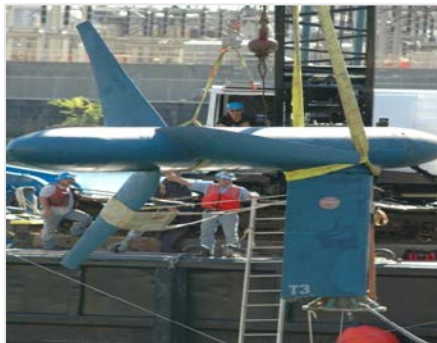
Turbines being lowered to underwater position
