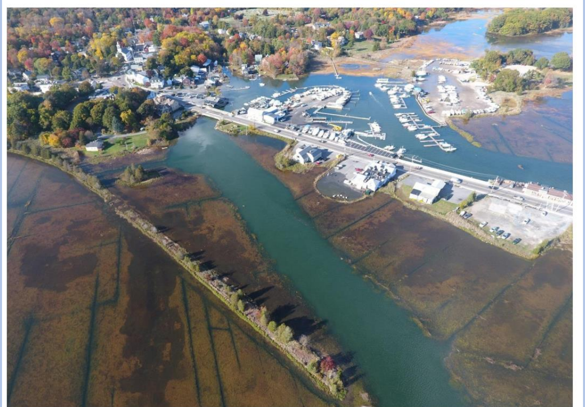
Essex Causeway/Main Street and businesses showing inundation from the Essex River. Photo credit: Abby Manzi, DeRosa Environmental
