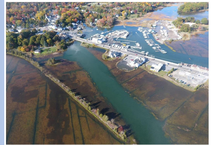
Essex Causeway/Main Street and businesses showing inundation from the Essex River. Photo credit: Abby Manzi, DeRosa Environmental
