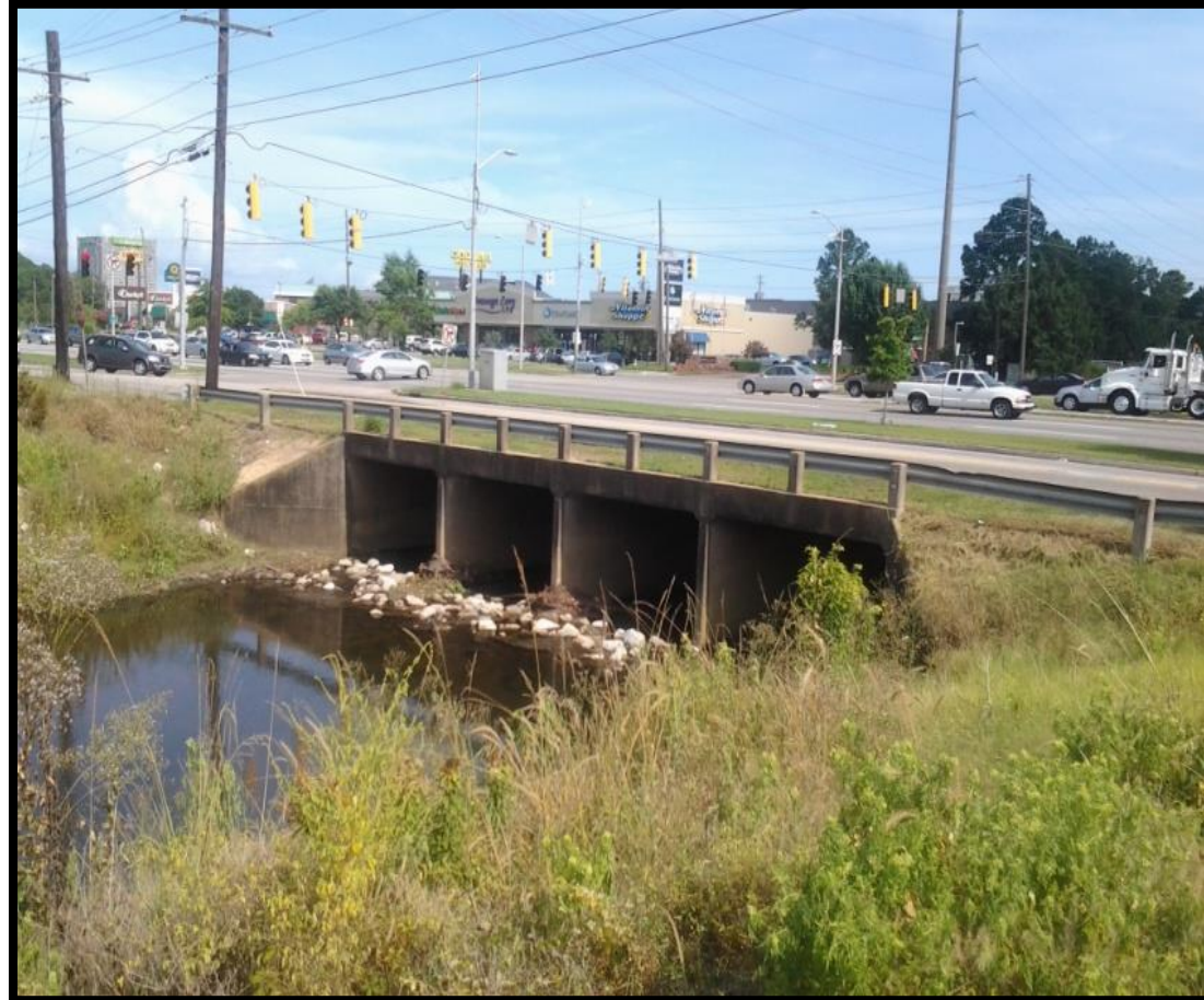
Photo: Culvert under Airport Boulevard (Mobile, AL)
