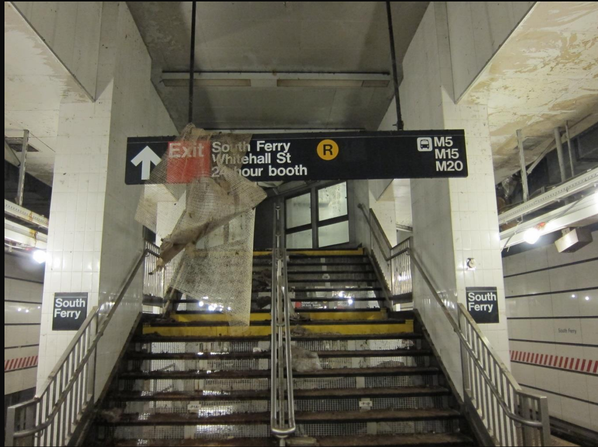
South Ferry Subway Station, Manhattan December 12, 2012
