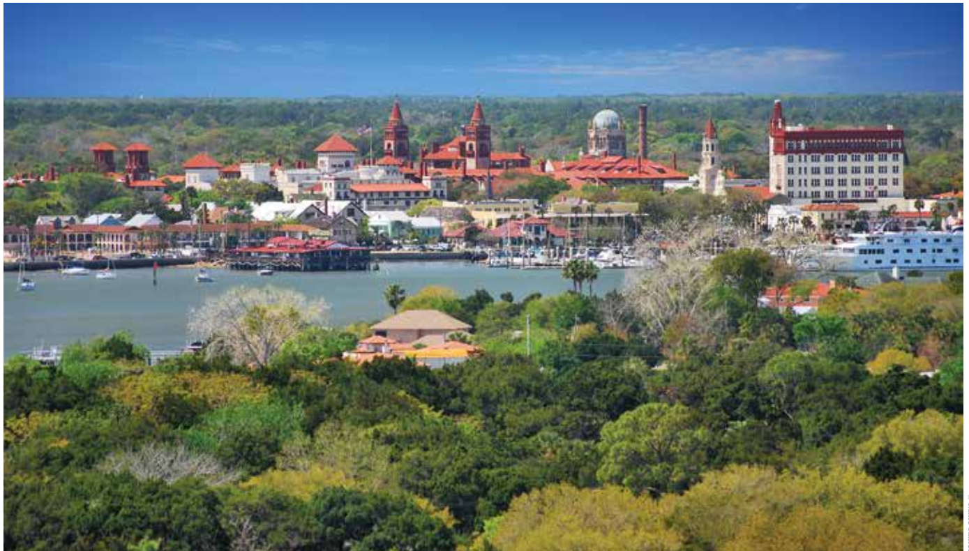
Sea level rise, worsening storm surges, erosion, and coastal flooding threaten landmarks in the nation’s oldest city. Established in 1565 as a Spanish fort, St. Augustine, FL, was the seat of Spanish rule in North America for 200 years.
