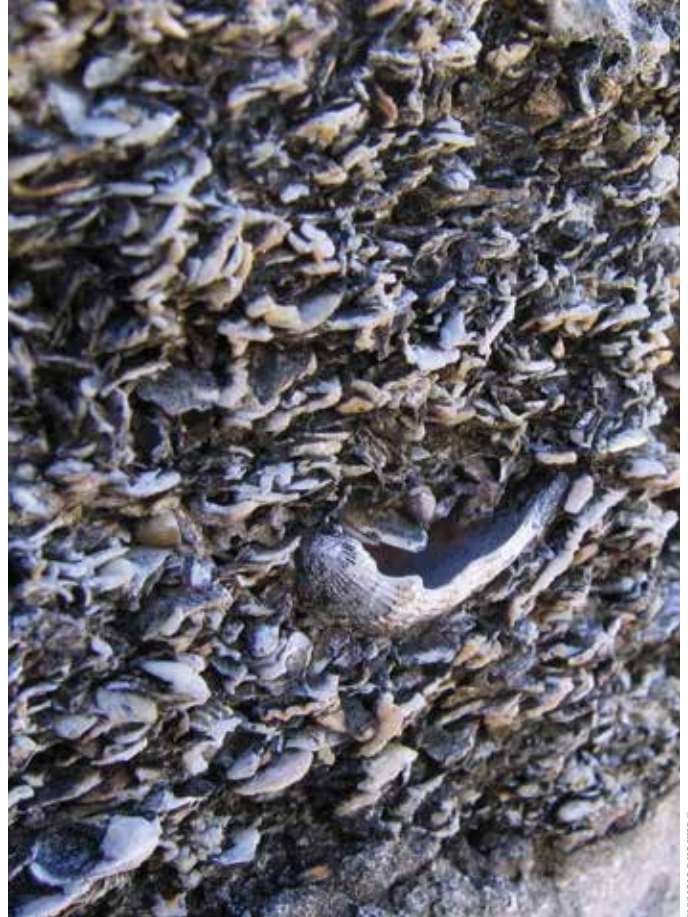
This close-up illustrates the coquina construction used at Castillo de San Marcos. The ocean's constant pounding meant the wall required reinforcement, and the National Park Service has taken steps to create a living seawall to protect the historic coquina wall.
