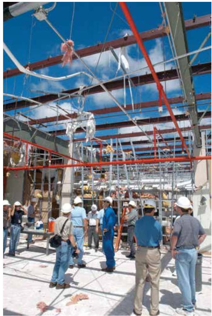
Members of a hurricane assessment team observe the damage to the roof of the Thermal Protection System (TPS) Facility at Kennedy Space Center after Hurricane Frances (2004). The facility, which created the TPS tiles, blankets, and all the internal thermal control systems for the space shuttles, was almost totally unserviceable after losing approximately 35 percent of its roof.
