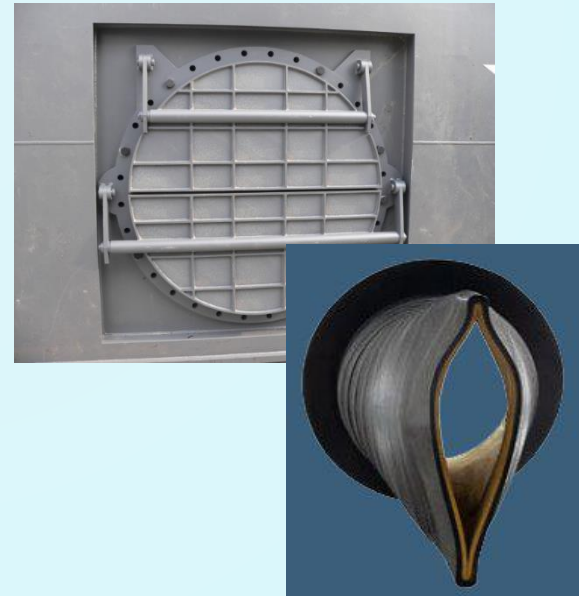
Coffer Dam protecting Market House, Flap Valve & Rubber Duckbill Valve
