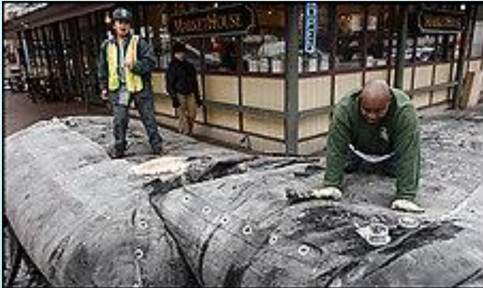
Coffer Dam protecting Market House, Flap Valve & Rubber Duckbill Valve
