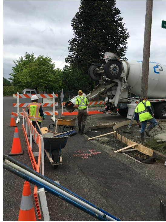
Pavement and ADA ramps
