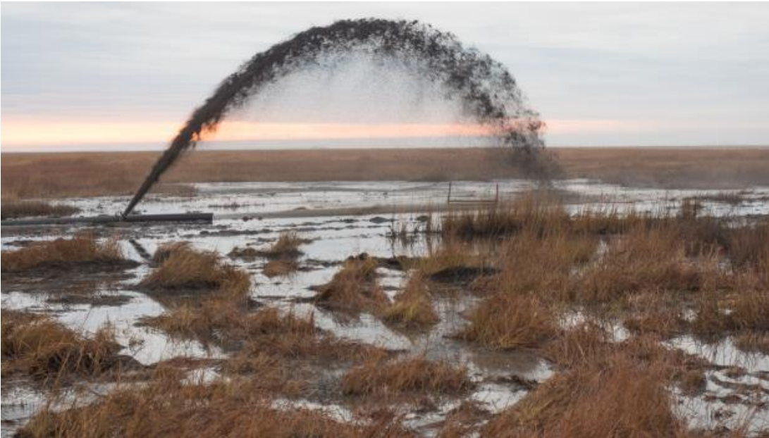
Thin layer placement of dredged sediment (source: https://usfwsnortheast.wordpress.com/2017/08/16/a-bottom-up-boost-for-coastal-habitat/ )
