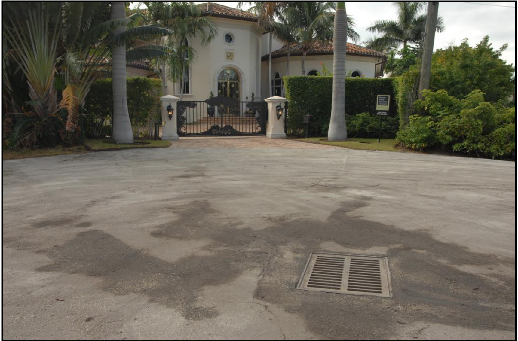
Storm drain located in cul de sac
