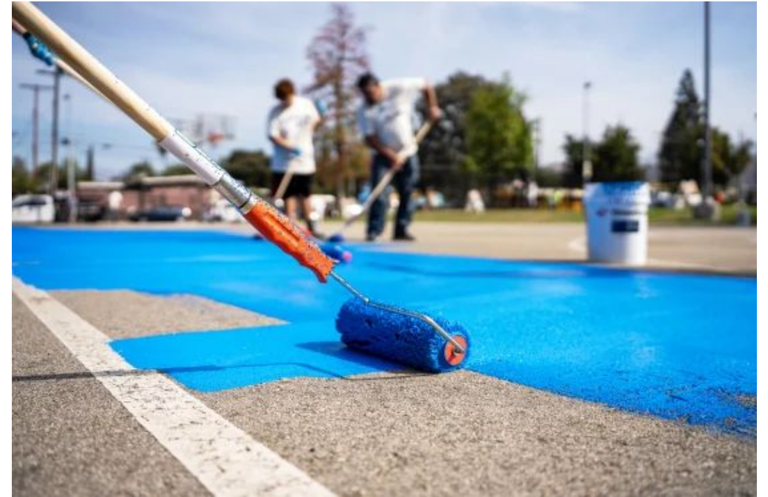
Solar reflective paint coating in Los Angeles Image Credit: GAF
