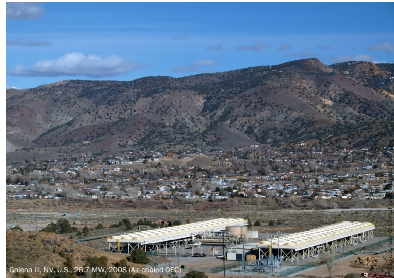
Galena III, NV, U.S., 26.7 MW, 2008 (Air-cooled OEC)
