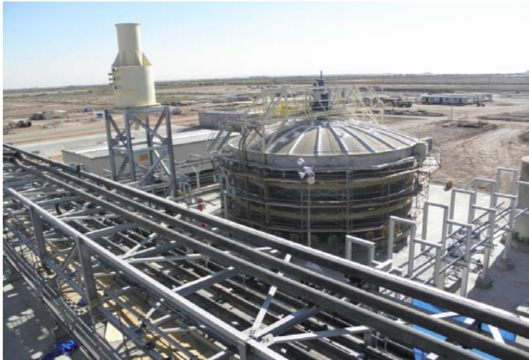
Galena III, NV, U.S., 26.7 MW, 2008 (Air-cooled OEC)
