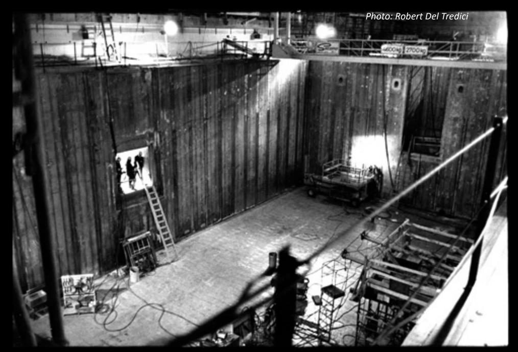
Irradiated fuel must be cooled for years by circulating water in a spent fuel pool.
