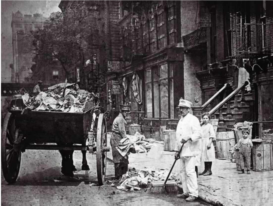
An early image of the sanitation department collecting trash, circa late 1890s. Photo courtesy DSNY.
