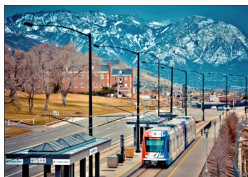
Salt Lake City's new light rail line
