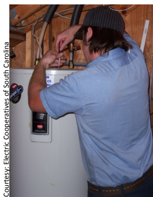
Insulating a water heater
