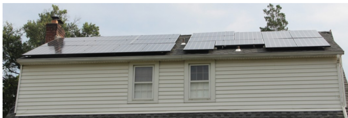
David's new solar installation is up and running
