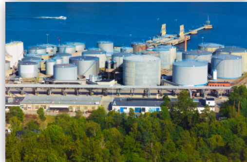
Fuel storage facility in Stockholm, Sweden.
