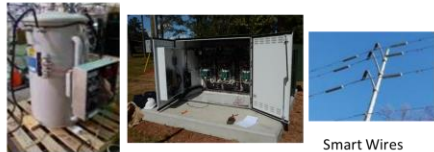
7.2 kV 50 kVA Hybrid Transformer 13 kV 1 MVA Modular Transformer
