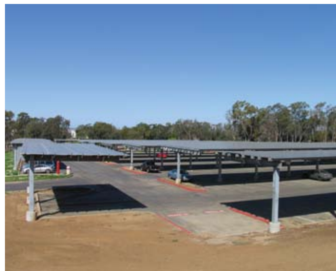
Photovoltaic installation at California State University, Dominguez Hills
