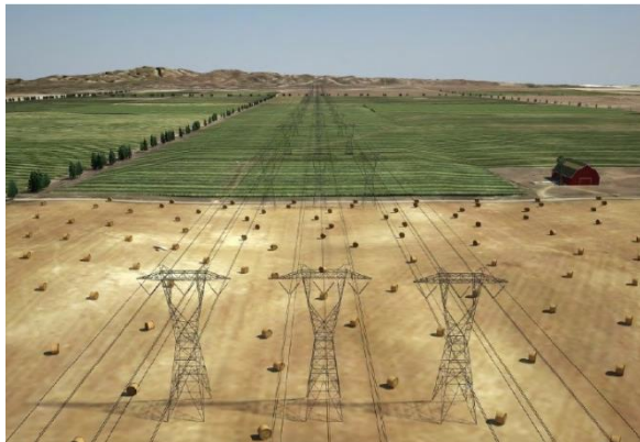
Three 500 kV lines
