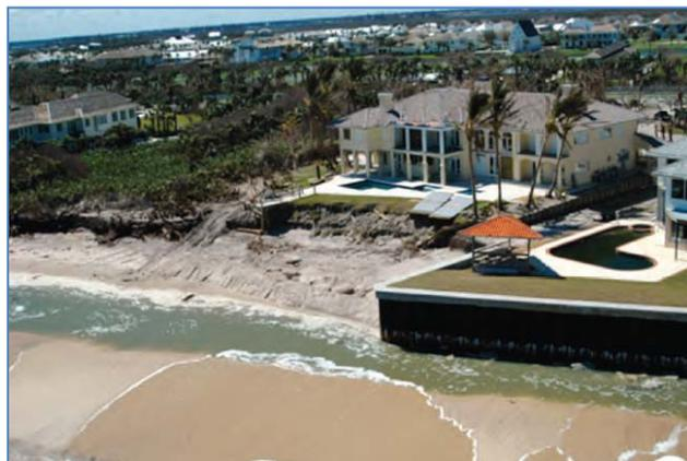
**Sea Walls (Dothan, Alabama)** The sea wall reflects wave energy and exacerbates erosion on the adjacent properties.
