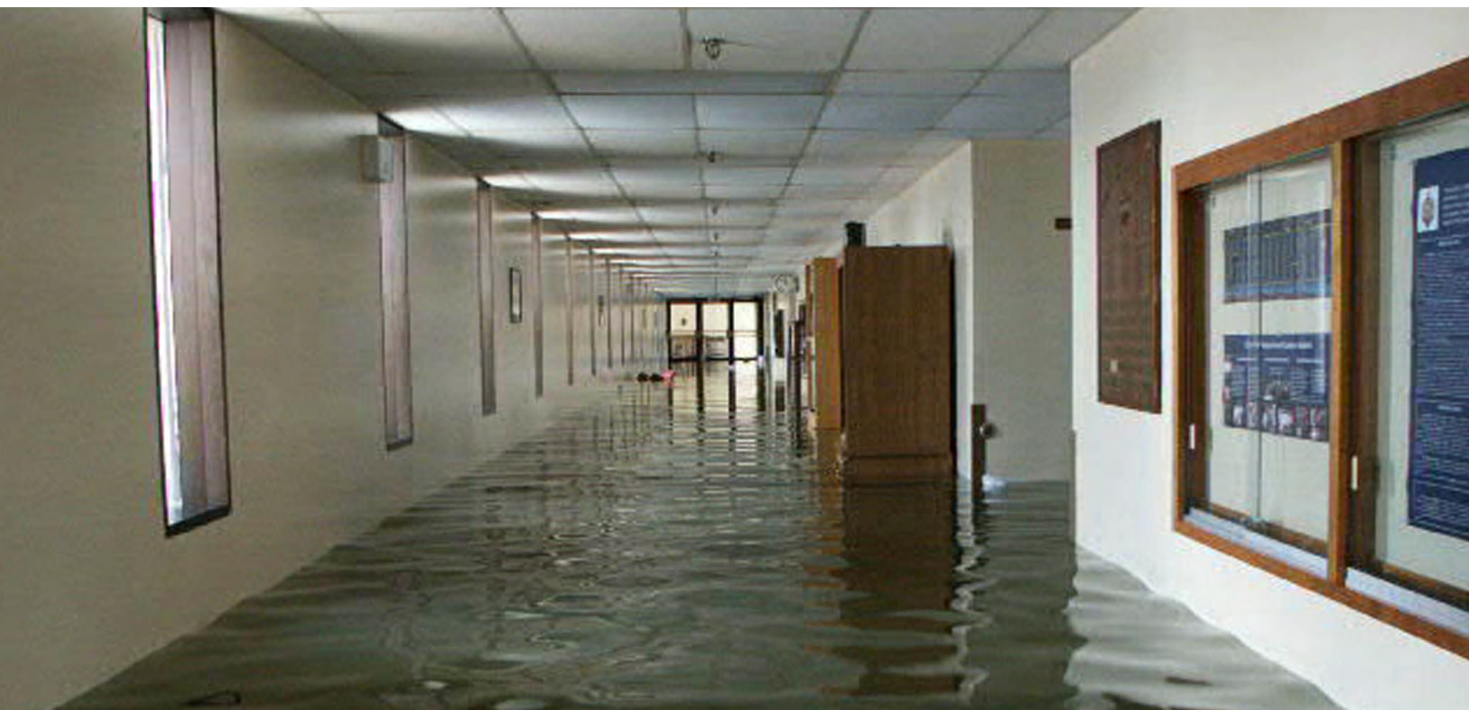
Floodwaters from storm surge caused by hurricane Isabel fills a corridor at the U.S. Naval Academy. September 2003. US NAVY
