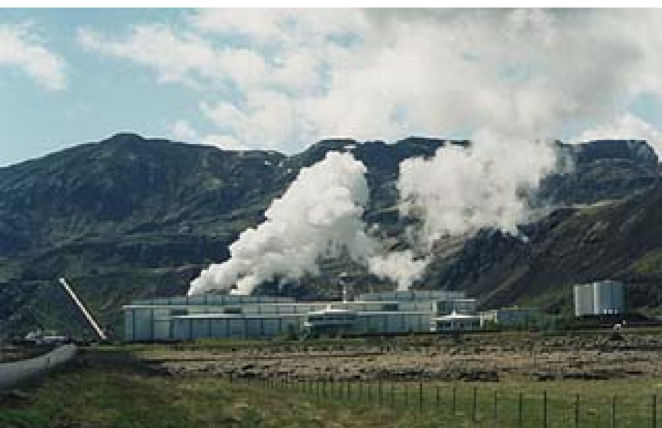
Geothermal Power: Nesjavellir Power Plant, Iceland; 90 MW
