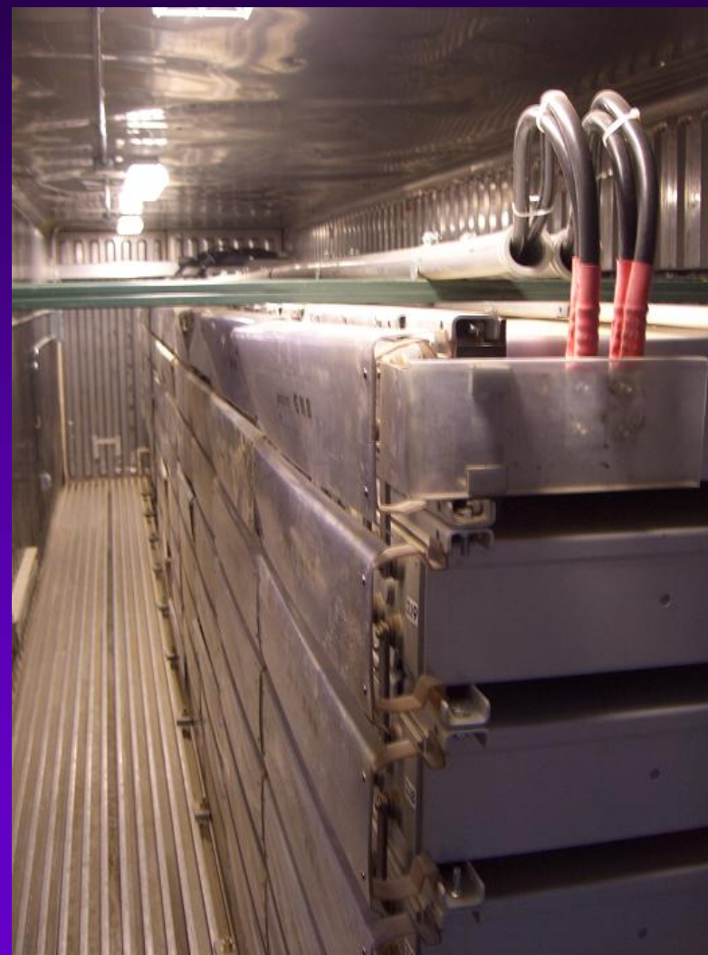
Batteries 3MW Total
