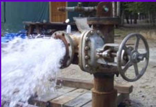
Geothermal Wells Provide Hot Water (~165F)
