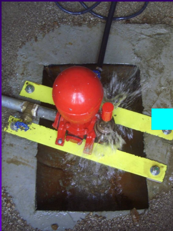
Water Ram pumps water from nearby creek (~1200gpd)
