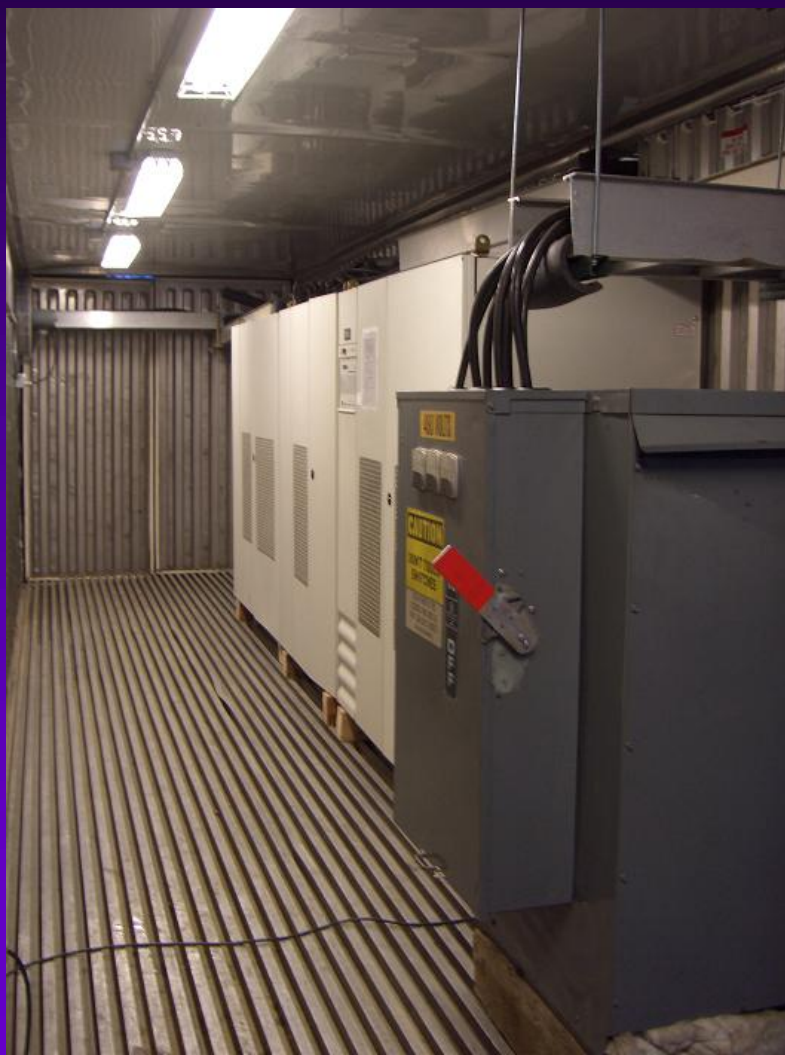
UPS System (MGE)
