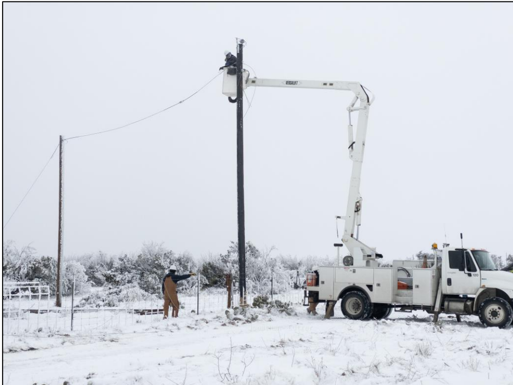
A crew works to restore power in Pecan Mott, TX on Feb 17 2021. Photo: Jonathan Cutrer (Flickr).
