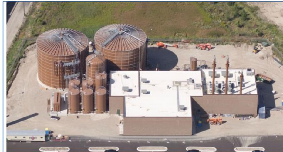
Photo 4: Food waste-to-energy biodigester facility, Forest County Potawatomi Community Renewable Generation, LLC
