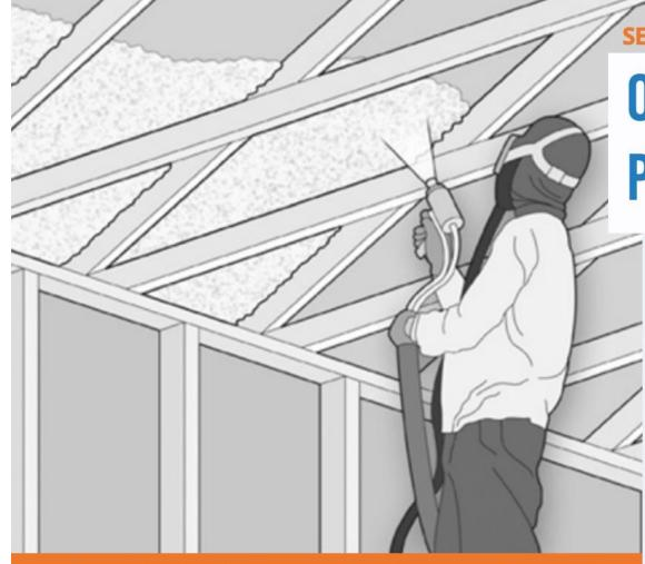
In the application of spray polyurethane foam, petrochemicals are reacted and create plastic envelopes around buildings.
