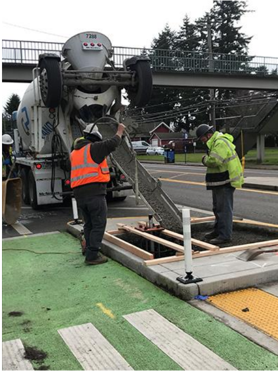
Traffic signal pole footing
