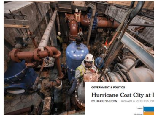
Workers this week replacing pumps at the Bay Park sewage...
