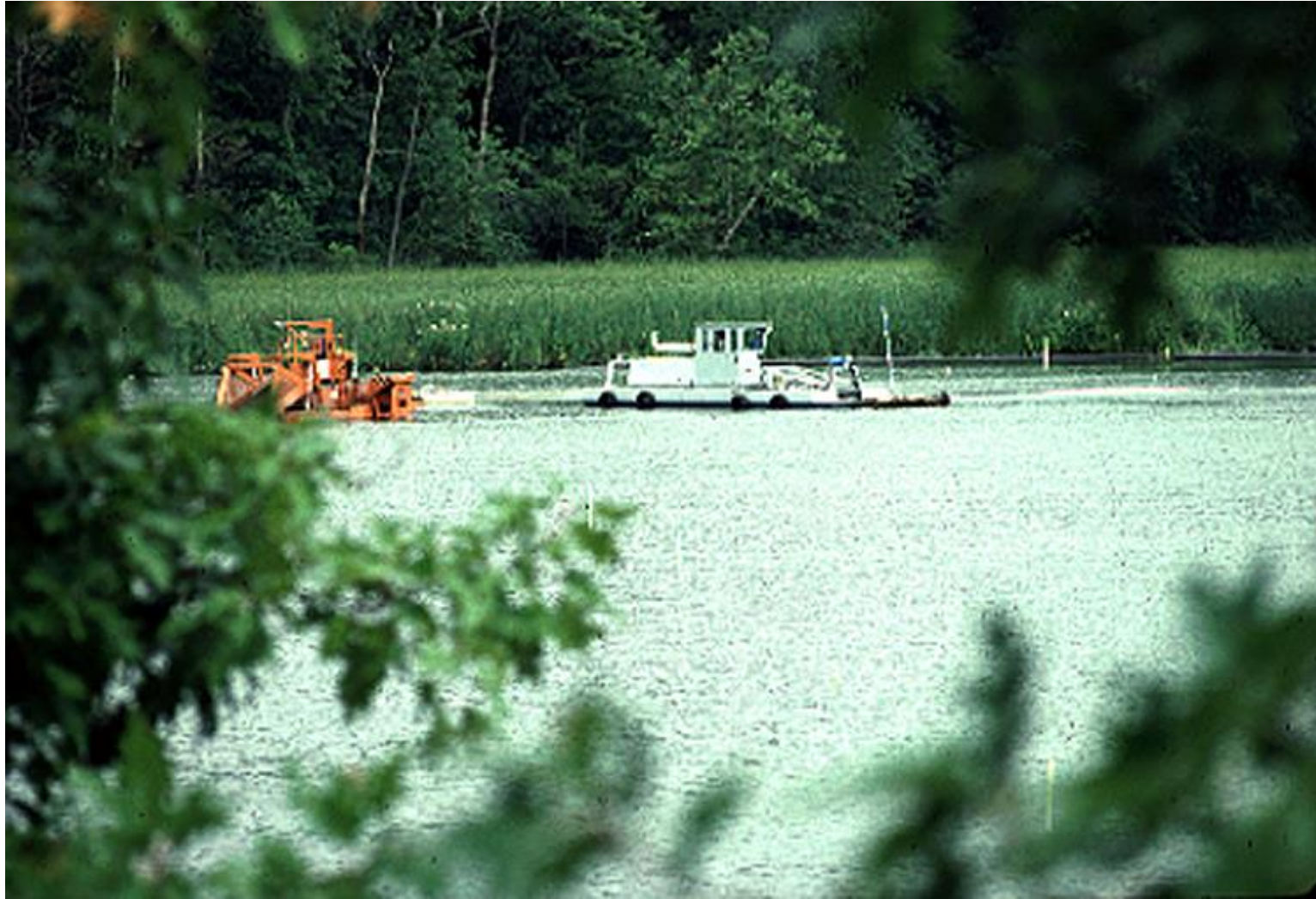
Dredging of Open Cove to Depth of 30 cm
