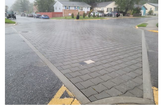
Intersections (Permeable Pavers)
