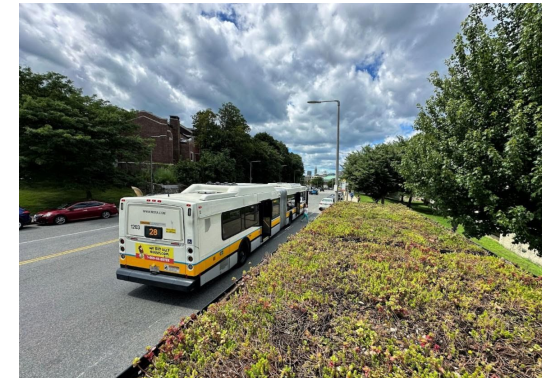
Bus Shelters (Green Roofs)
