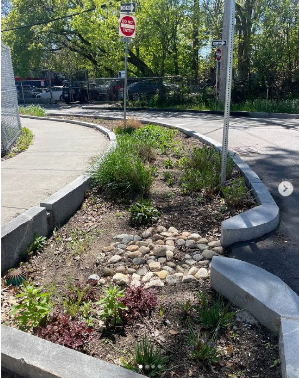
Green infrastructure curb extension in Dorchester neighborhood of Boston, MA
