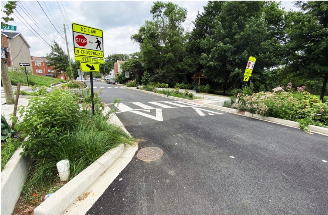
Retrofitted intersection with stormwater retention and traffic calming in DC Image Credit: Toole Design
