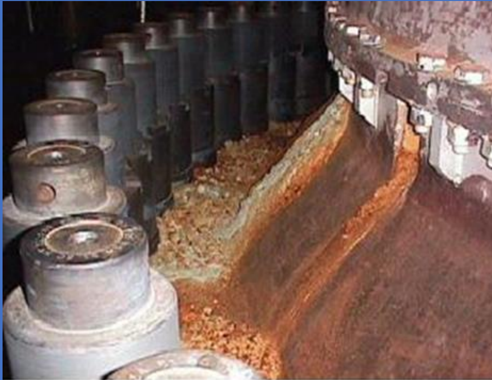
Red Rusty Boric Acid Deposits on Vessel Flange (12RFO)
