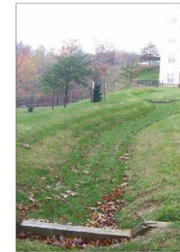
Grass drainage swale
