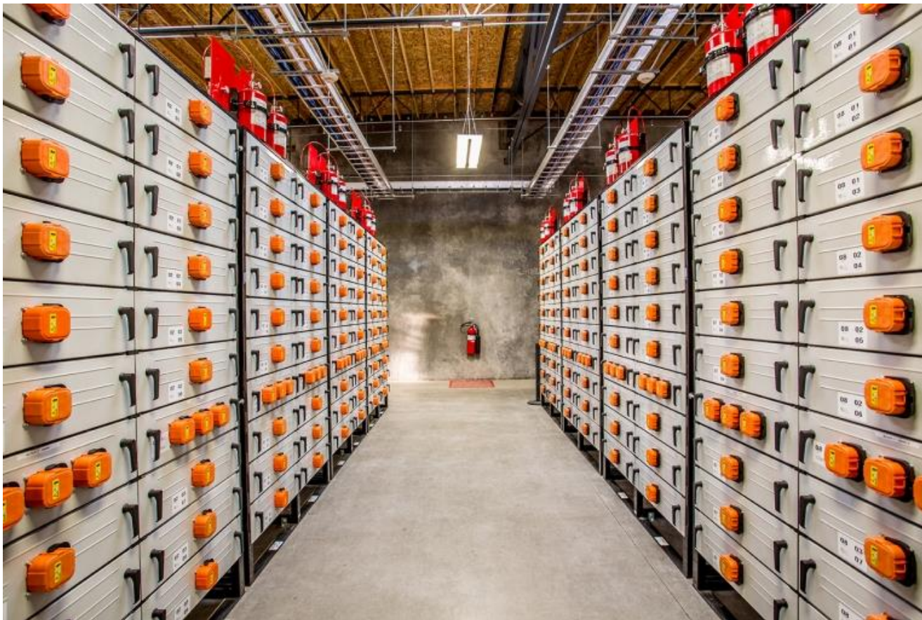
5 MW Energy Storage System at the Salem Smart Power Center in Salem, OR
