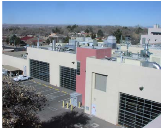
The Ford Utilities Center
